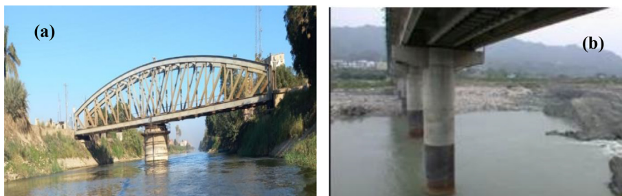
Fig. 1 Photographs for bridges with circular piers: (a) single circular pier; (b) multi-circular piers.
